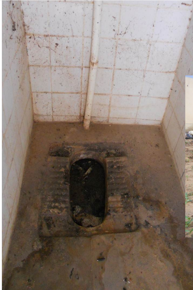
Clogged latrines (built 2010) in Meskine Health Care Centre, Cameroon
