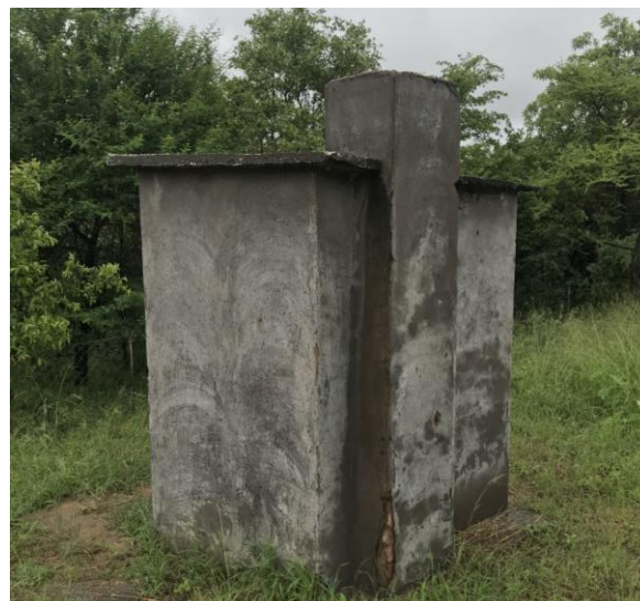
Figure 1. Sanitation facility at a rural health centre in Zimbabwe.
