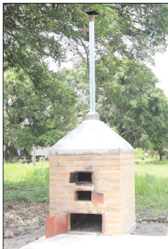
New Incinerator. Built by World Vision, Mutzing, Markham District, Morobe Province (photo by Bernice Sarpong)
