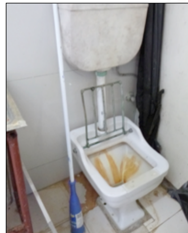
Adequate disposal of wastewater from cleaning is required such as this deep sink for bucket slops (photo by Rhonda Clement, WaterAid PNG)
