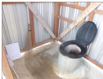
Interior of VIP toilets, Lemikot Nursing School, New Ireland Province (photo by Penny Dutton)
