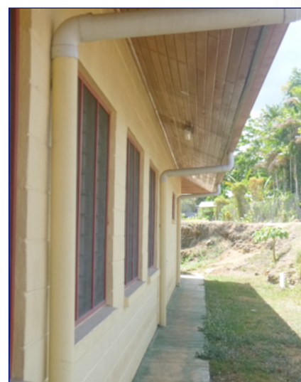
Roof runoff. Rainwater can be captured for storage or diverted to drains (photo by Penny Dutton)
