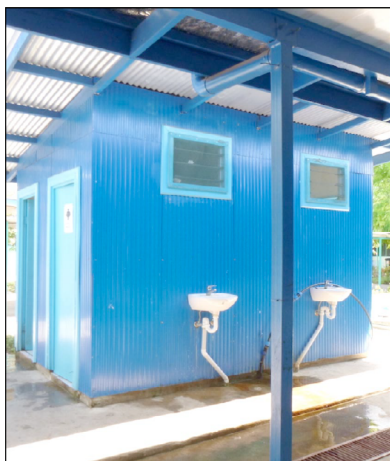
Cleaning and maintenance of toilets is important
