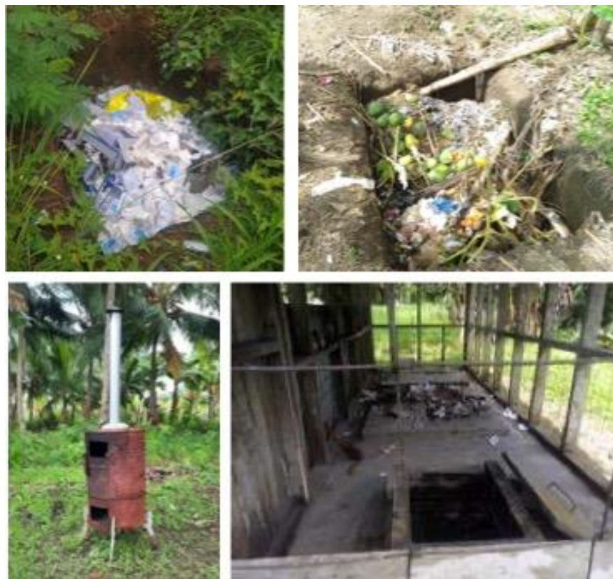
Figure 27 Waste Management Facilities in HCFs
