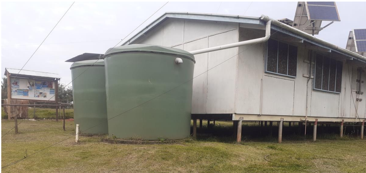
Figure 11 Rainwater tanks at RSHC
