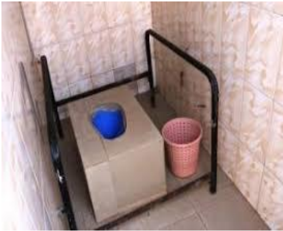
FIGURE 8: DESIGNS OF SANITATION FACILITIES FOR PEOPLE WITH SPECIAL NEEDS
