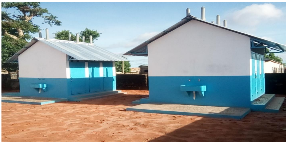
FIGURE 6: VENTILATED IMPROVED PIT LATRINES
