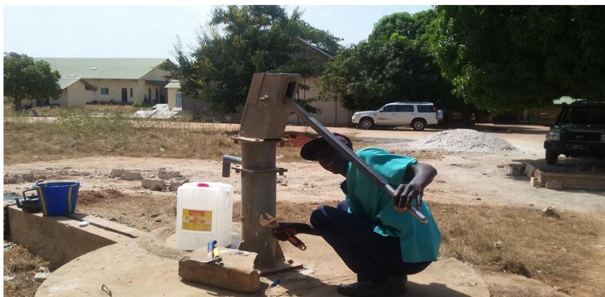
FIGURE 3: MAINTENANCE OF HAND PUMP AT SOMA H/C
