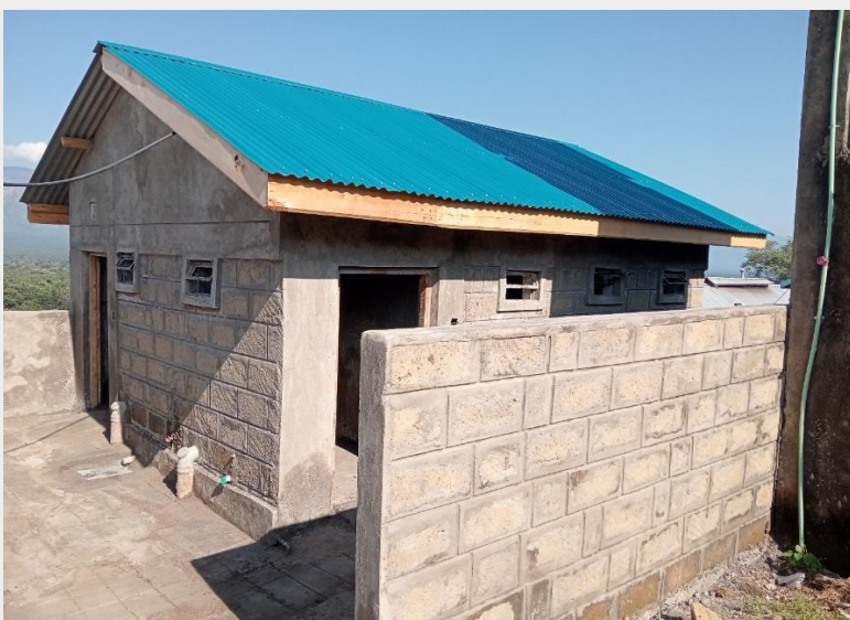
Photo of Inclusive Washrooms and Bathrooms constructed
