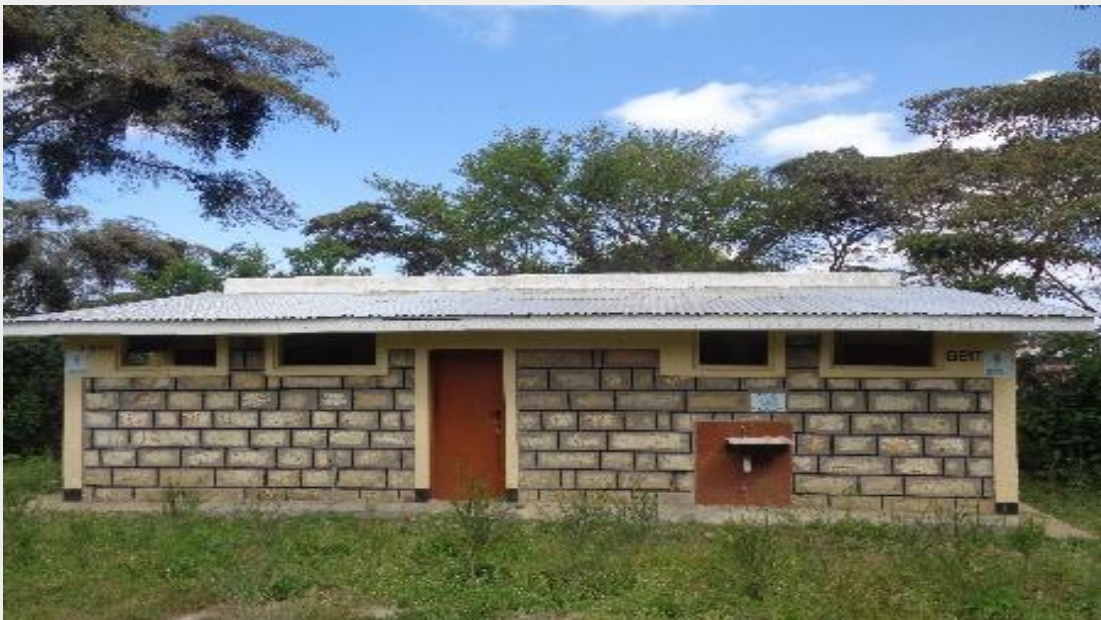
New toilets at the facility
