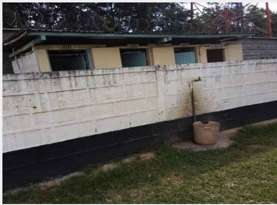
Old pit latrines
