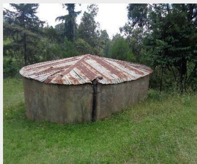
Previous water storage tank
