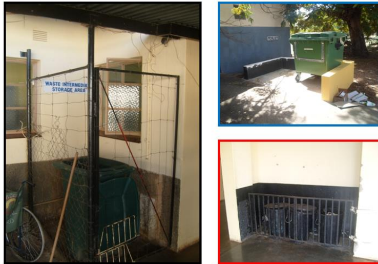
Figure 41 Intermediate storage for waste
