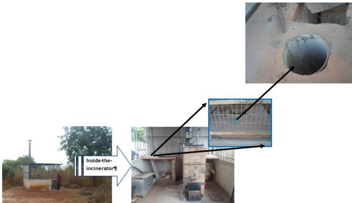
Figure 64 Pathological Waste pit at Incinerator sites
